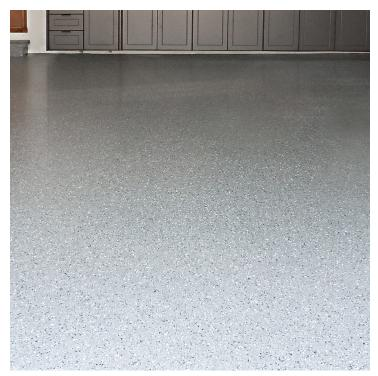
Professionally applied epoxy or other polyurea finishes can make your floor look better than new. Proper preparation is key to professional applications... cracks are repaired and the surface is ground smooth prior to applying the coating. Color choices are almost limitless to match any decor.
